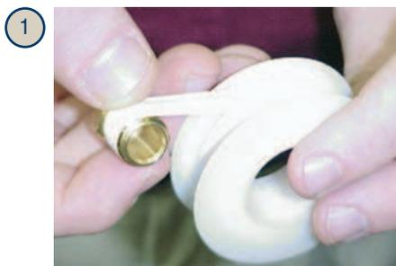
Apply 1½ to 2 wraps of PTFE tape, starting one or two threads from the lead edge, in a clockwise direction. For 316 stainless steel, be sure to use stainless grade tape.
